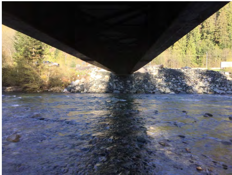
Right Bank Abutment when facing downstream
