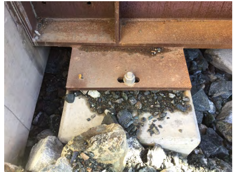
Right bank bearing
